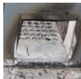
b: Removable steel grate in the Leo double pot stove
